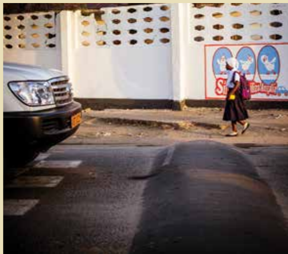
An example of cheap but effective traffic calming implemented as part of the SARSAI programme
