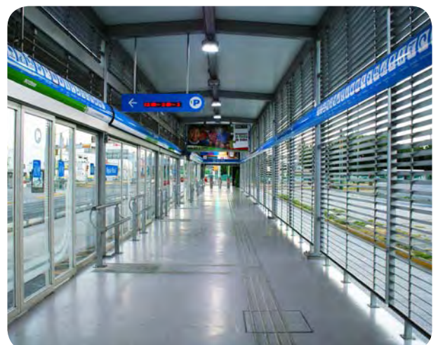
Interior of a BRT station, Guadalajara, Mexico © Colectivo Ecologista Jalisco
