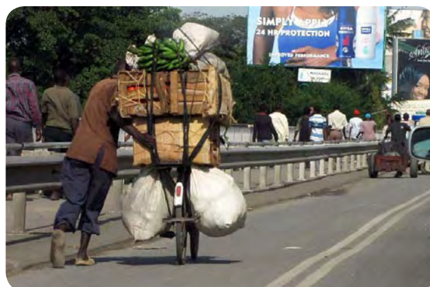
Widened hard shoulder can be used as a cycle lane for crossing a bridge © UNEP
