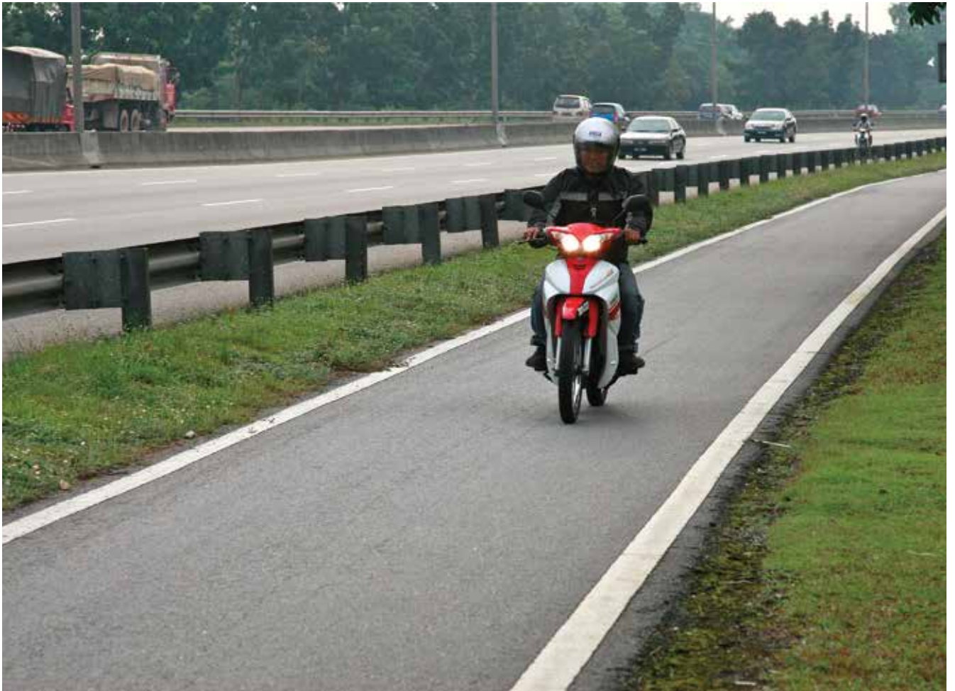
This separated motorcycle lane in Malaysia is a good example of 'forgiving' infrastructure
