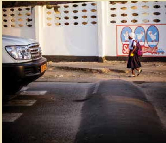
An example of cheap but effective traffic calming implemented as part of the SARSAI programme
